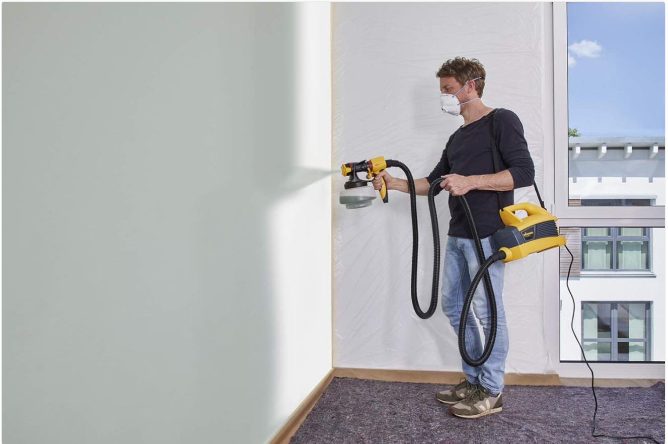
Image 4: A user demonstrating the application of paint to an interior wall using the WAGNER W 690 FLEXiO system, highlighting proper technique and distance.
