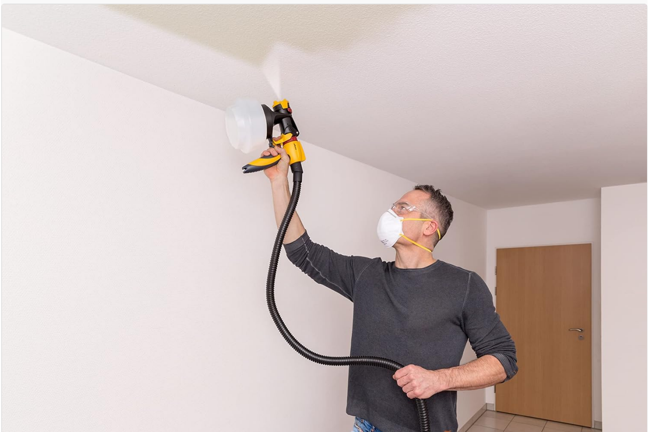
Image 5: A user applying paint to a ceiling with the WAGNER W 690 FLEXiO, illustrating overhead spraying technique for large
