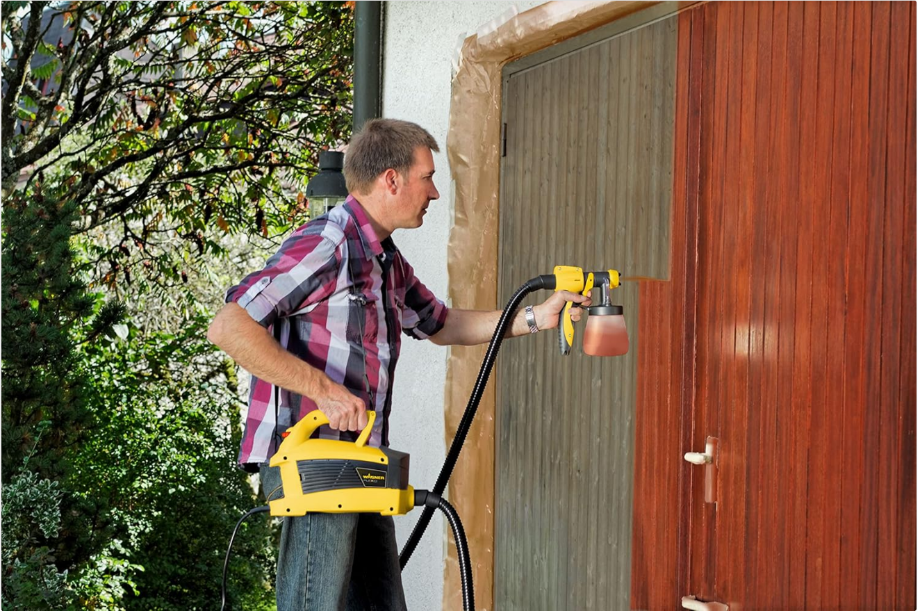
Image 8: A user spraying a wooden garage door, demonstrating the application of wood protection or glaze with the WAGNER W 690 FLEXiO.
