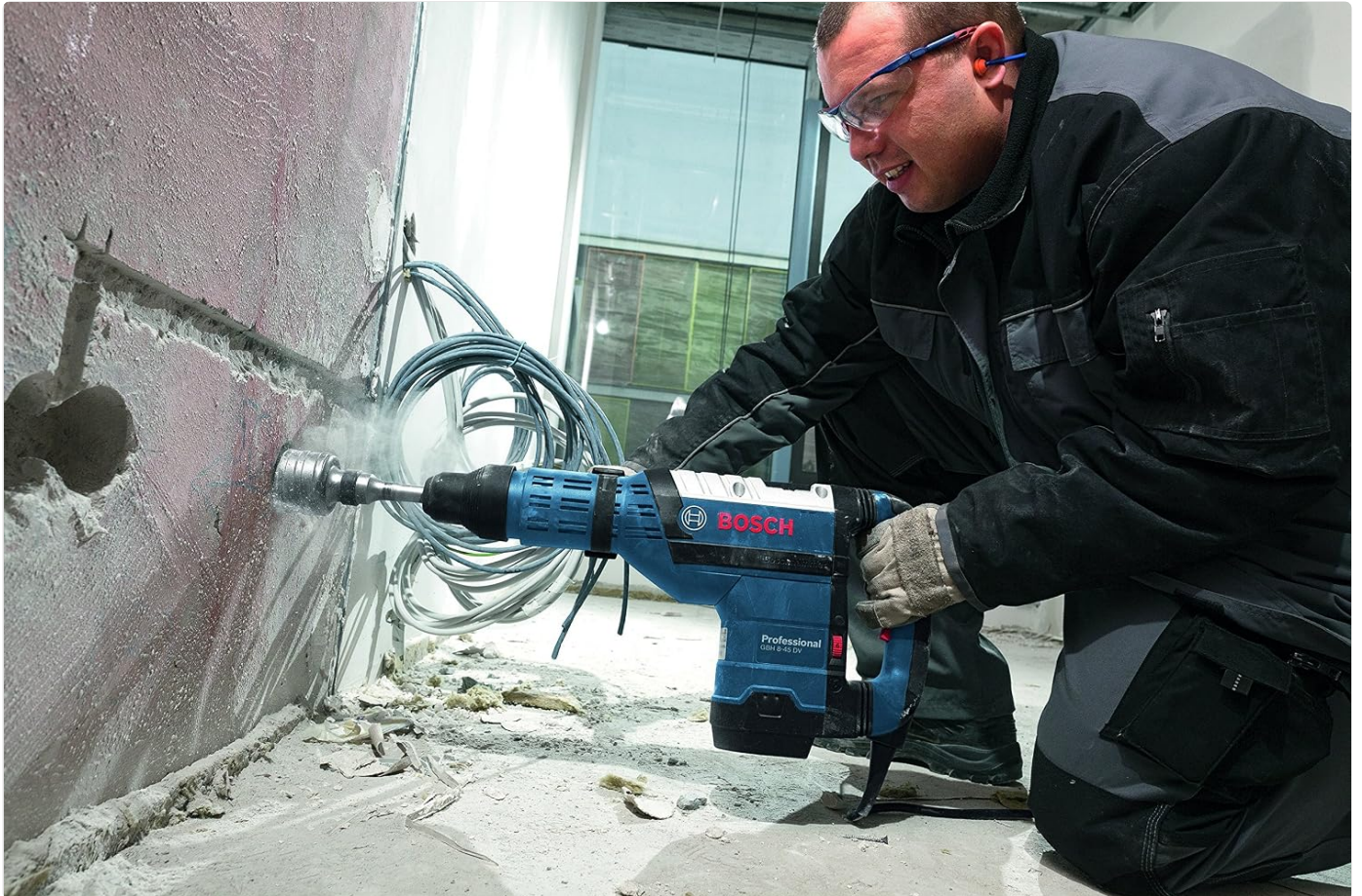
Image: A worker operating the Bosch GBH 8-45 DV rotary hammer to drill a large hole into a concrete wall, demonstrating its application in construction.
