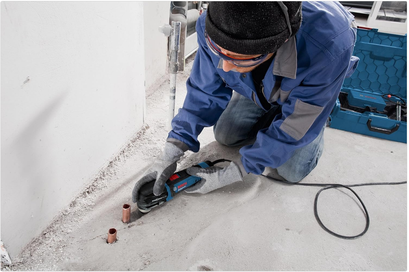
Figure 5.1: A professional using the Bosch GOP 30-28 Multi-Tool for precise cutting of a pipe near a floor surface.
