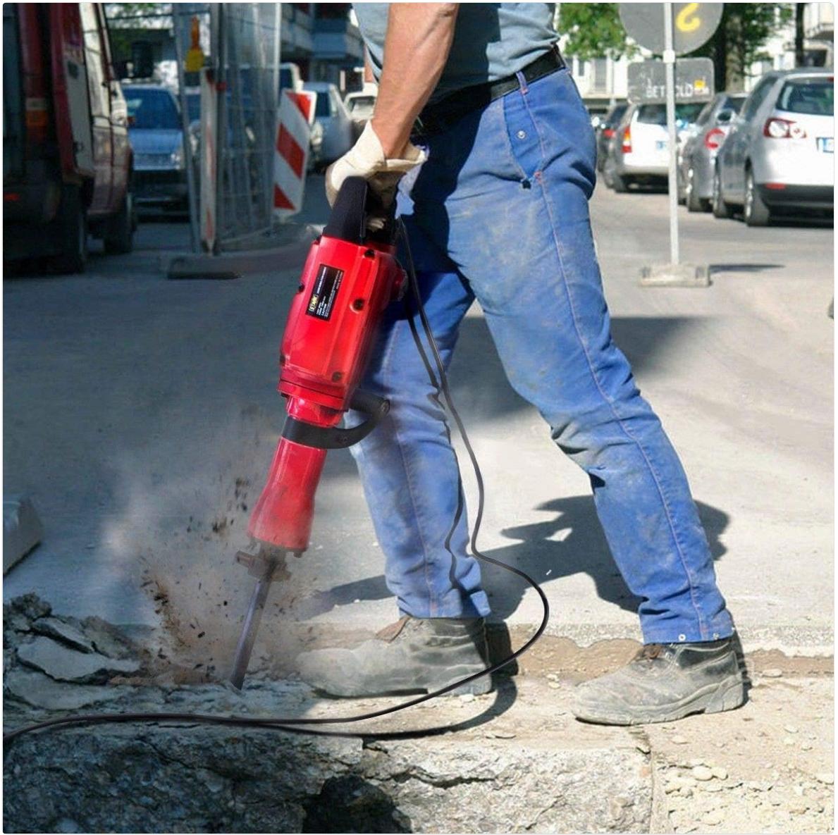
Image 6.2: The jack hammer in action on an outdoor concrete surface, demonstrating its application in breaking up pavement or other hard materials.
