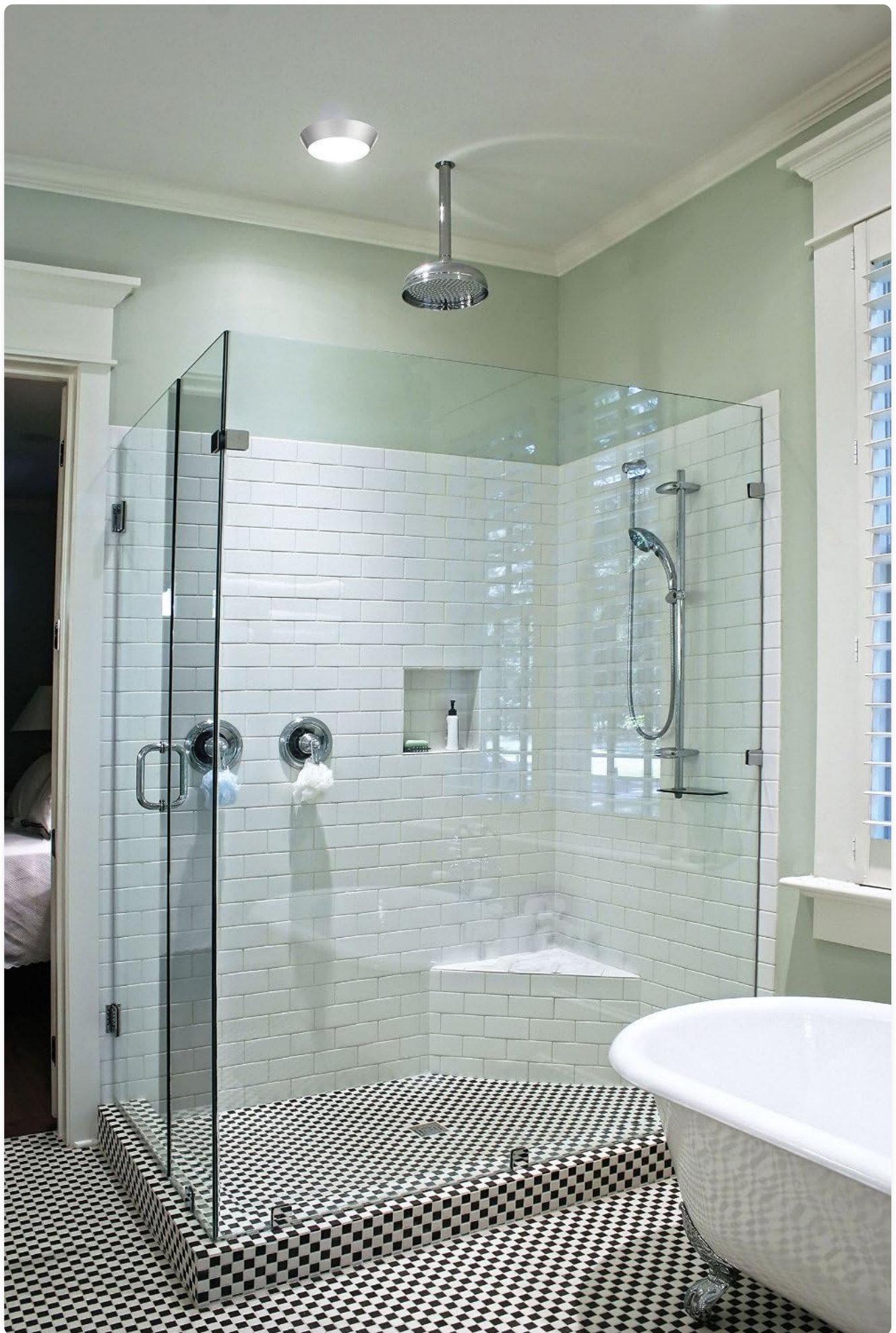
Figure 4: The fixture's damp listing makes it suitable for use in bathrooms, as shown here.
