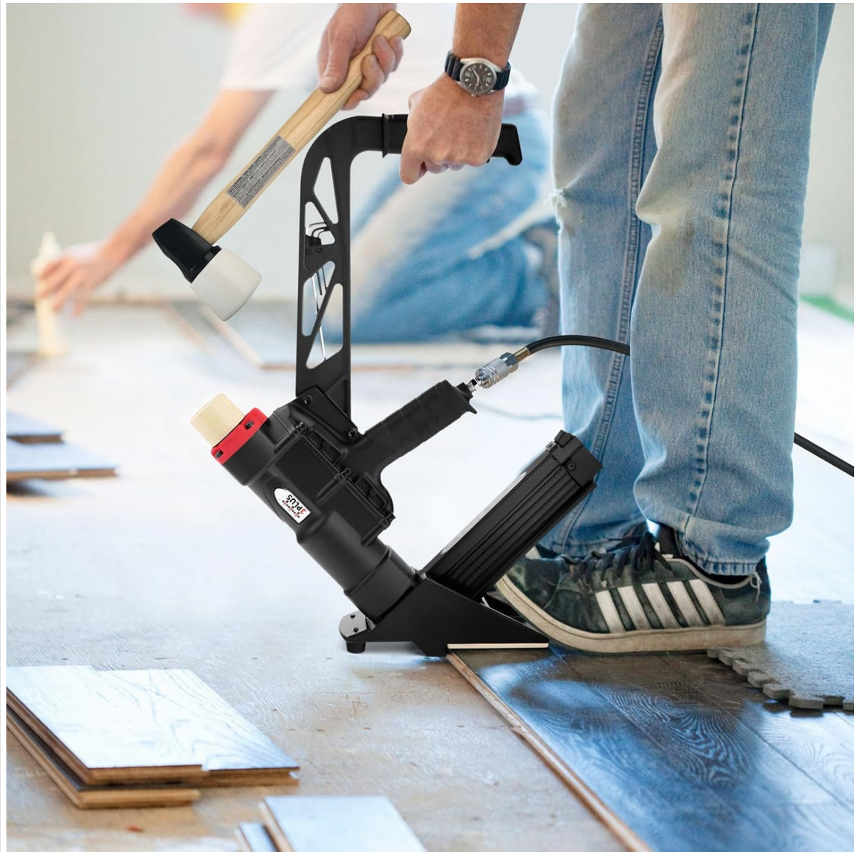
Figure 7: The flooring nailer/stapler in use, demonstrating proper positioning for driving fasteners into a hardwood plank.
