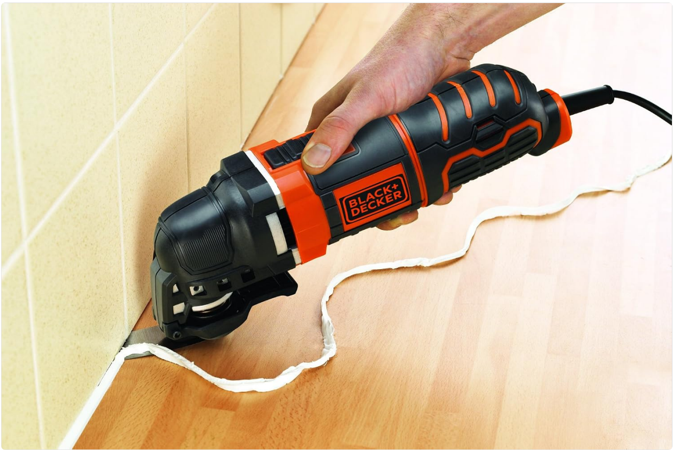
Figure 6.4: The multi-tool effectively removing old caulk or sealant from the edge of a floor, demonstrating its precision for detail work.
