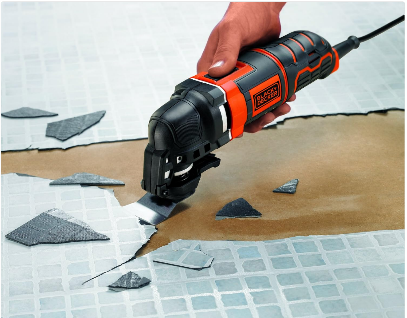
Figure 6.5: The multi-tool being used to scrape and remove old floor tiles or adhesive, showcasing its power for demolition and renovation tasks.
