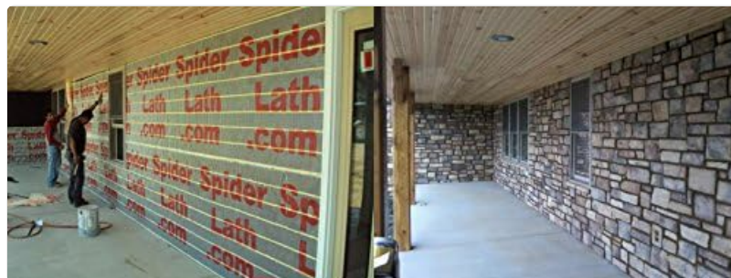
Image: An example of a finished exterior wall with stone veneer successfully applied over SpiderLath.
