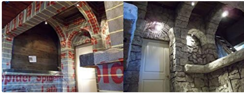
Image: A detailed view illustrating the self-furring mechanism, showing the 1/4 inch spacing behind and on top of the lath.
