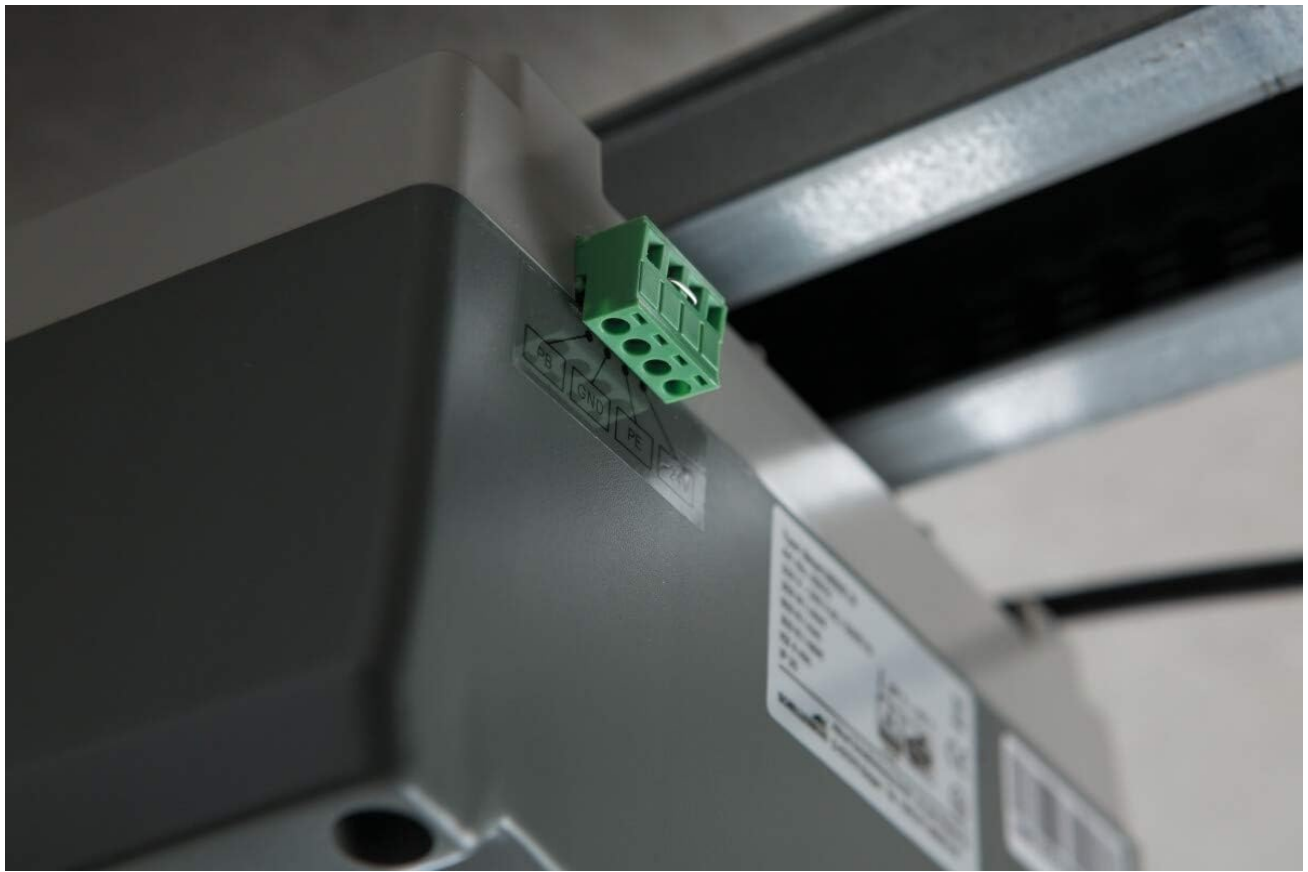
Image 5.2: Wiring terminal for optional external connections.
