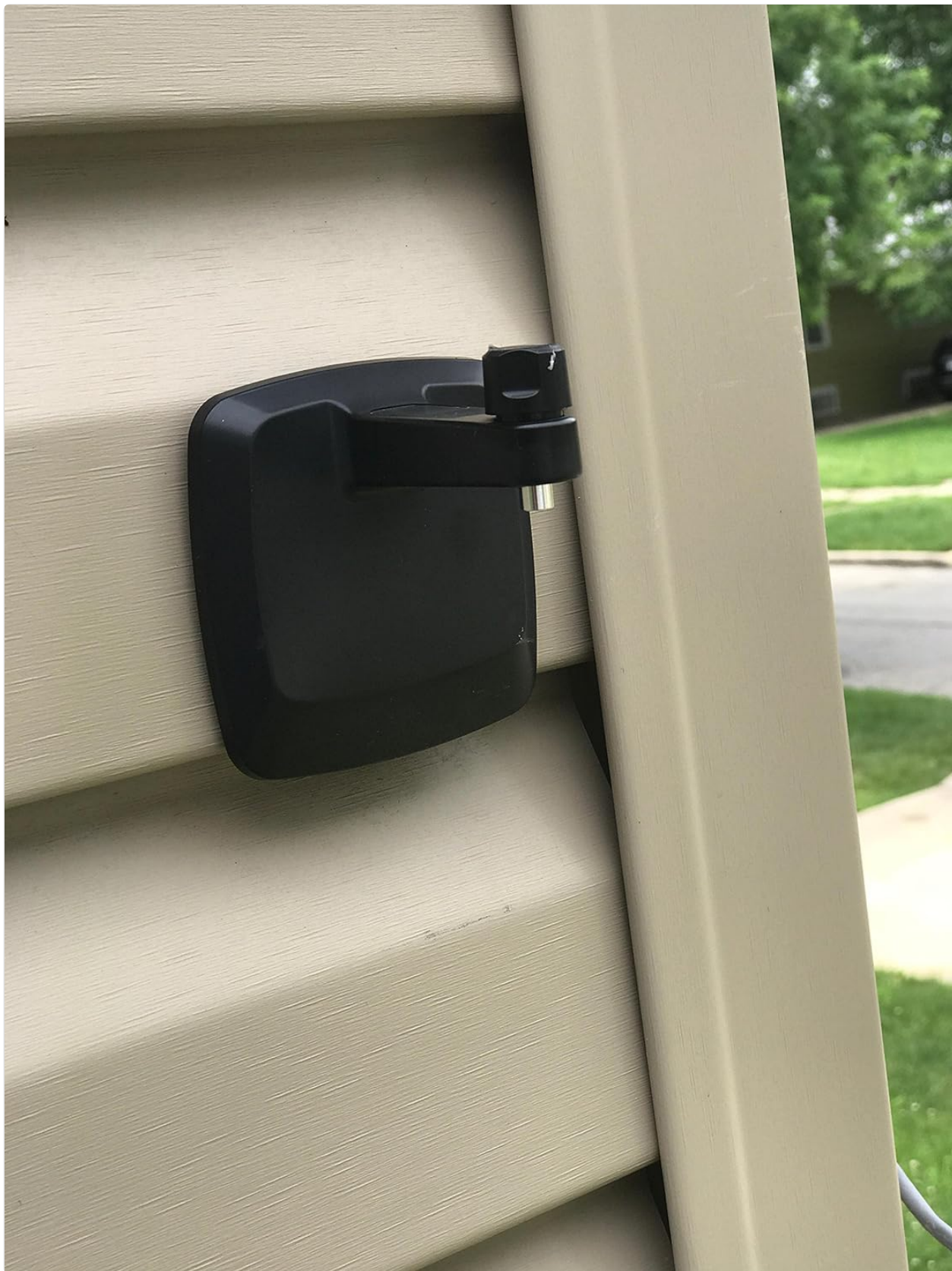
Figure 4.1: The ICamera2 securely mounted on exterior house siding, demonstrating outdoor installation.
