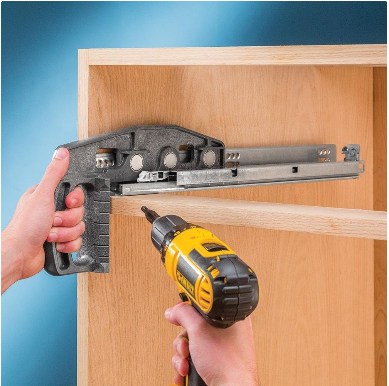
Image: A drill being used to drive screws through the jig's access holes, securing the drawer slide.
