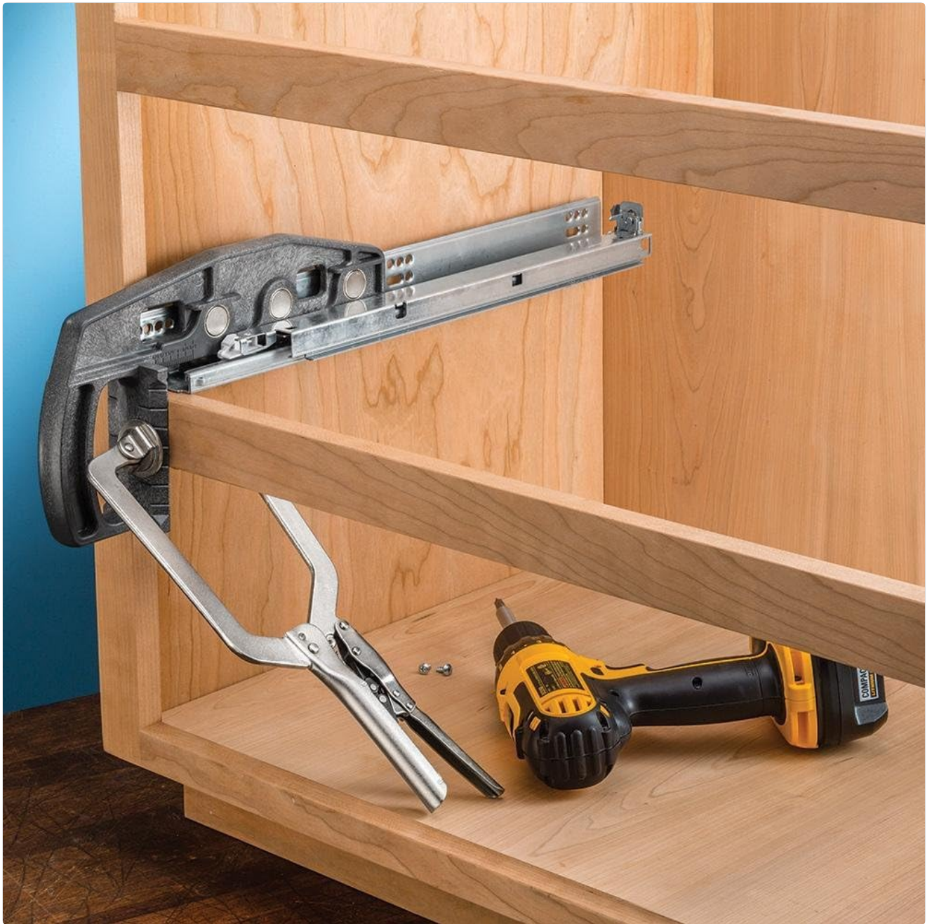
Image: The jig secured with a clamp, providing extra stability during the installation process.
