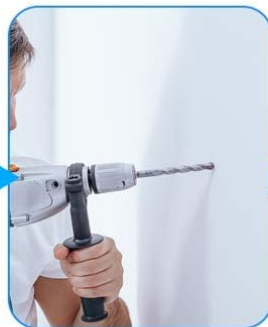
2. Drill a hole
