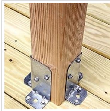
Image 4.4: A Simpson Strong-Tie post cap securely installed on a wooden deck, connecting a vertical post to the deck structure, with all fasteners in place.
