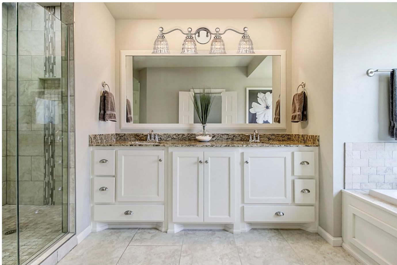
Image: Savoy House Birone 4-Light Vanity Bar installed above a bathroom mirror, showcasing its polished nickel finish and clear patterned glass shades.
