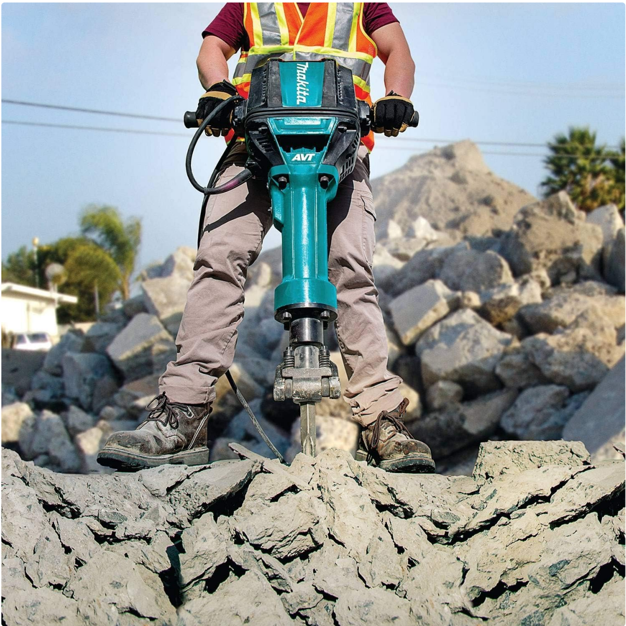
Close-up view of the breaker hammer's bit engaging with concrete.
