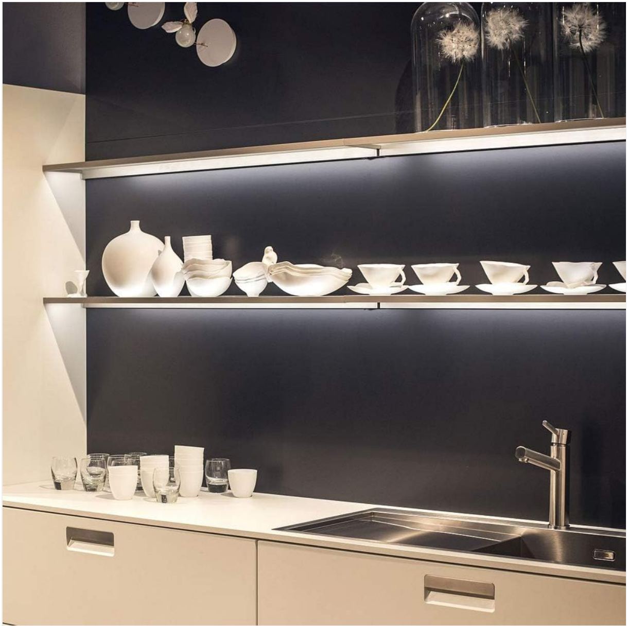
Image 5.3: Example of LED strip lights providing illumination under kitchen cabinets.
