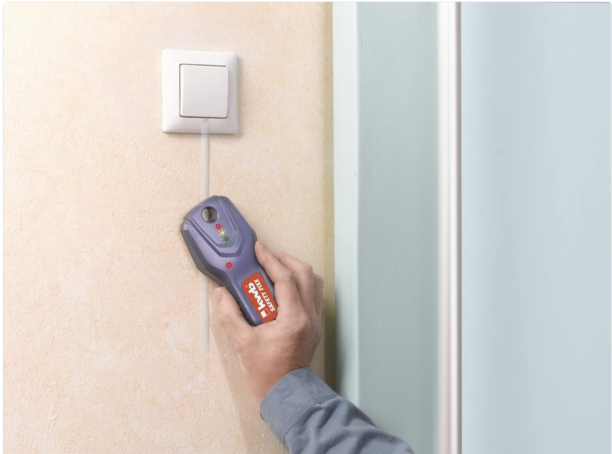
Figure 2: Detecting electrical cables near an outlet.
