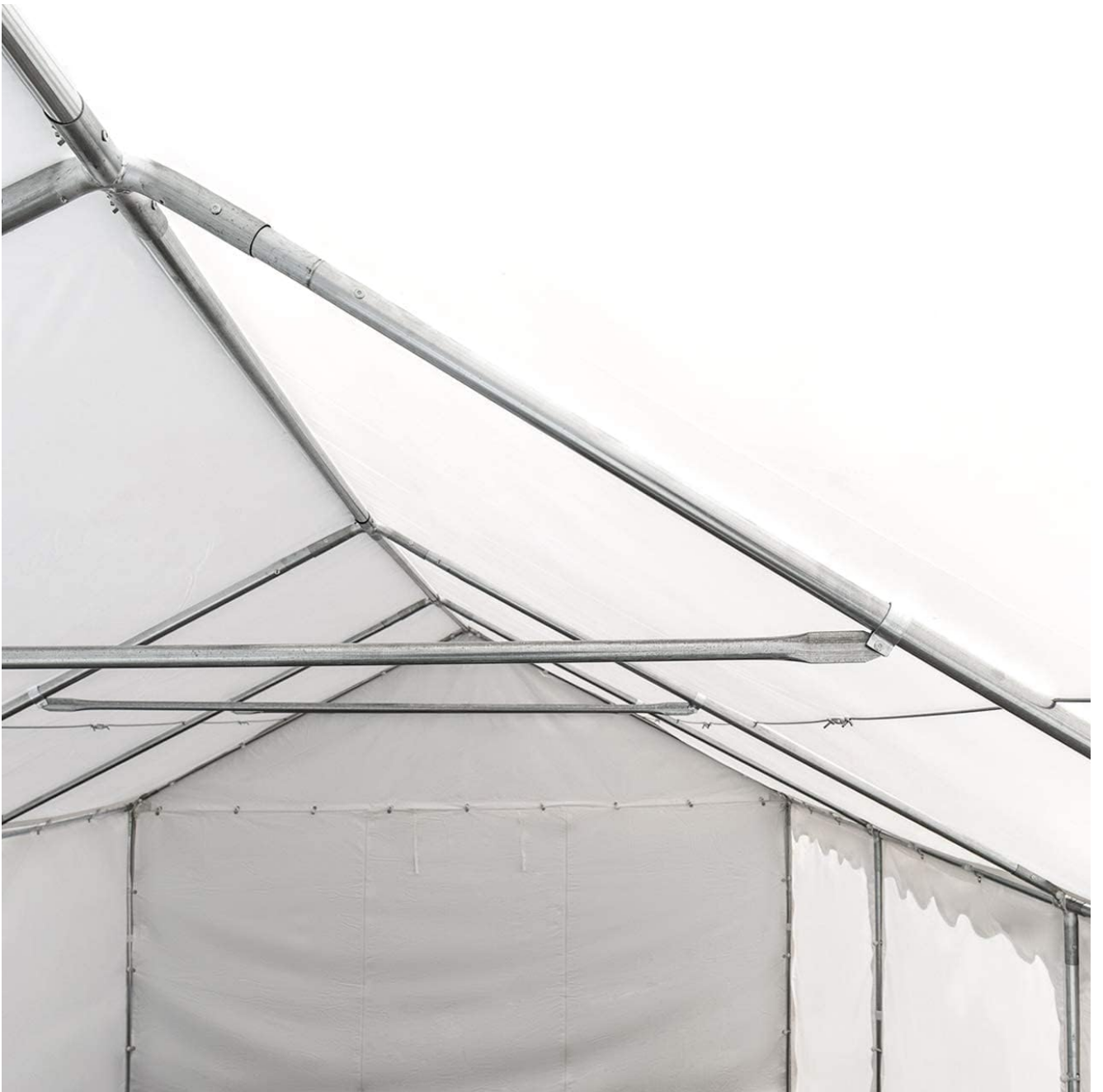
Image: View of the interior roof structure, showing the galvanized steel tubes and bolted connections.
