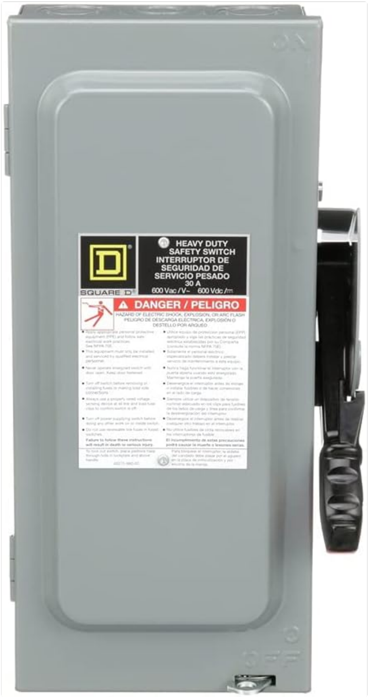
Figure 3.1: Front view of the Square D H361 Safety Switch, showing the main enclosure and operating handle.
