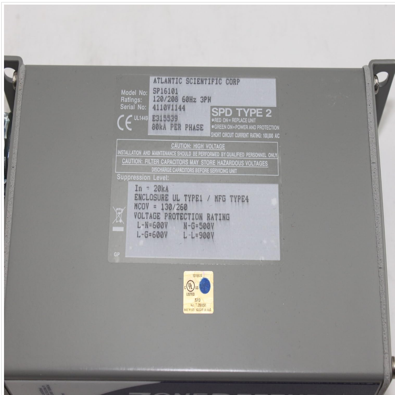
Image 1: Product Label. This image displays the product label of the Eaton Crouse Hinds Zone Defender Pro SP16101 surge protector. The label provides critical information including the model number (SP16101), electrical ratings (120/208 60Hz 3PH), serial number (4110V1144), UL listing (UL1449 E315509), SPD Type 2, 80kA per phase rating, and a short circuit current rating of 100,000 AIC. It also includes important safety warnings regarding high voltage and the need for qualified personnel for installation and maintenance. Suppression levels (In=20kA), enclosure type (UL TYPE1 / MFG TYPE4), MCOV (130/260), and Voltage Protection Ratings (L-N=600V, N-G=500V, L-G=600V, L-L=900V) are also visible.
