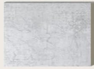
Concrete Wall (Anchor Required)
