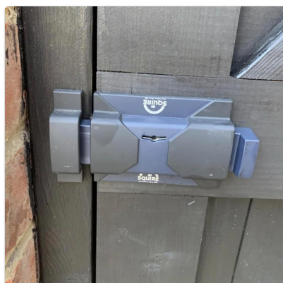
Image 10.1: Keybolt installed on a wooden gate.
