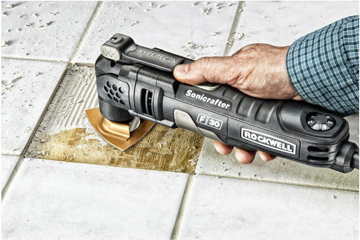
Image 5.6: The multi-tool with a scraping blade, effectively removing old adhesive or material from a surface.
