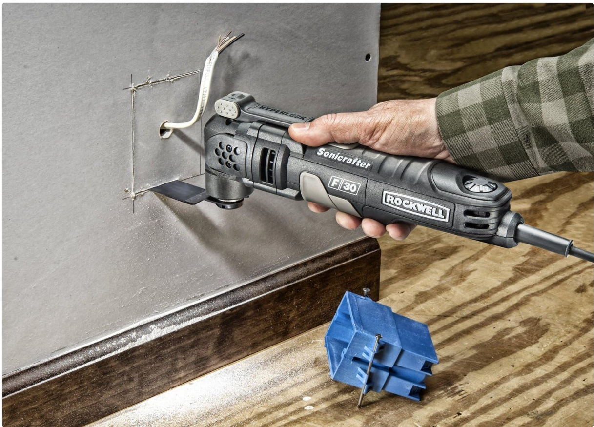
Image 5.4: The multi-tool making a precise cut in drywall to install an electrical box, showcasing its use in renovation tasks.
