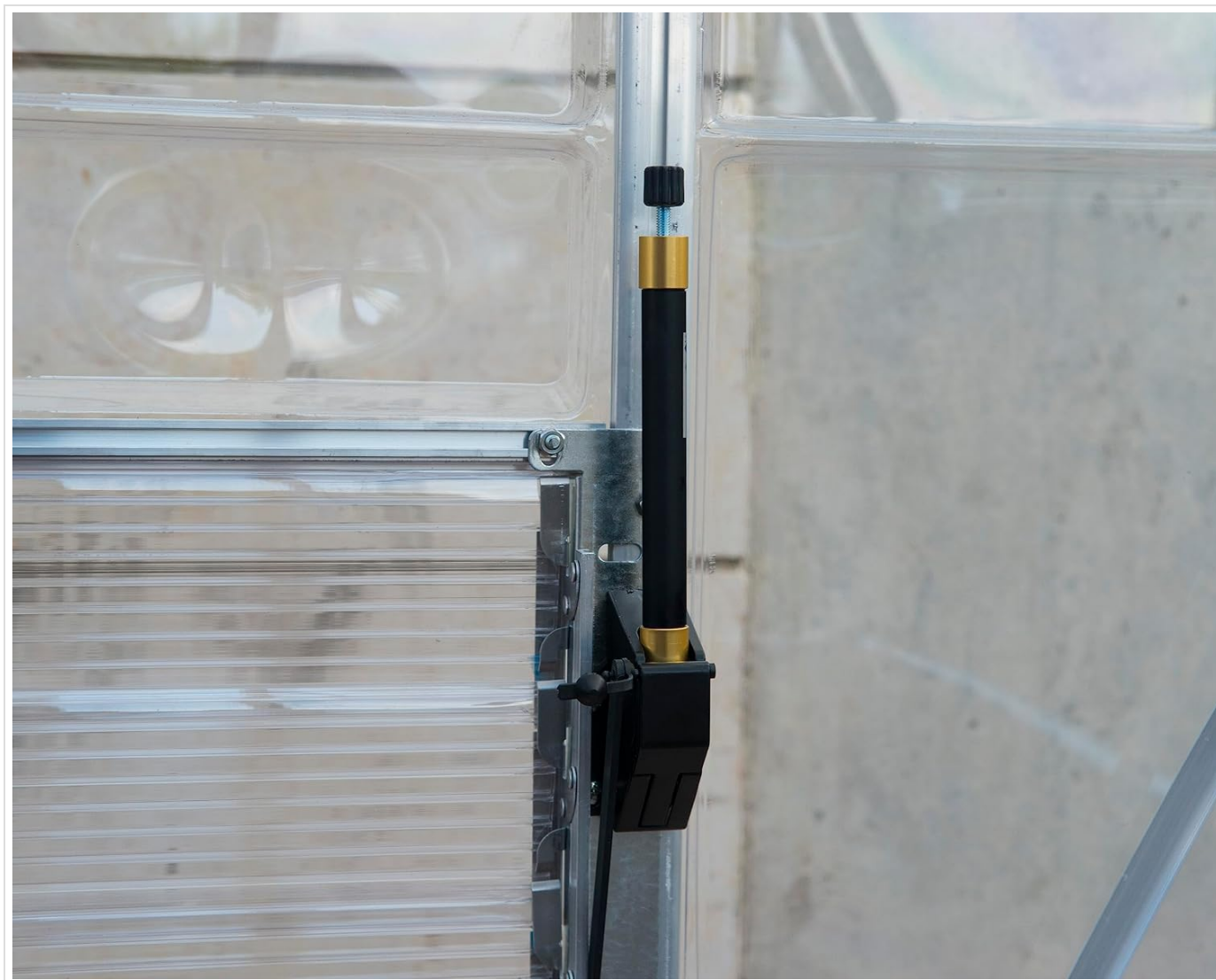
Figure 2: The automatic louver opener unit mounted to the greenhouse frame, with the louver in a closed position. The black cylinder and arm are visible, connected to the louver mechanism.
