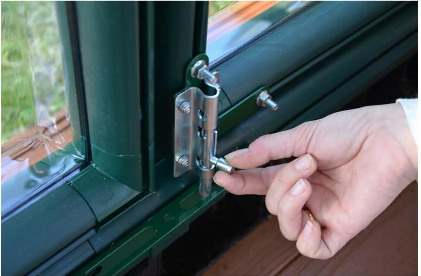
Figure 3: A hand securing a pin within the greenhouse frame, illustrating the simplicity of the Pin & Lock connection. It is recommended to secure the greenhouse to a concrete pad or heavy timber foundation for maximum stability.
