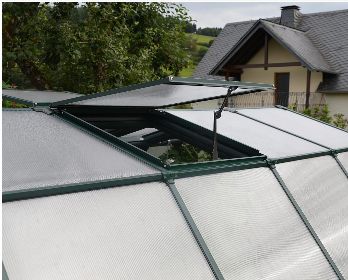
Figure 6: The roof vent in an open position, facilitating air exchange and temperature regulation within the greenhouse.
