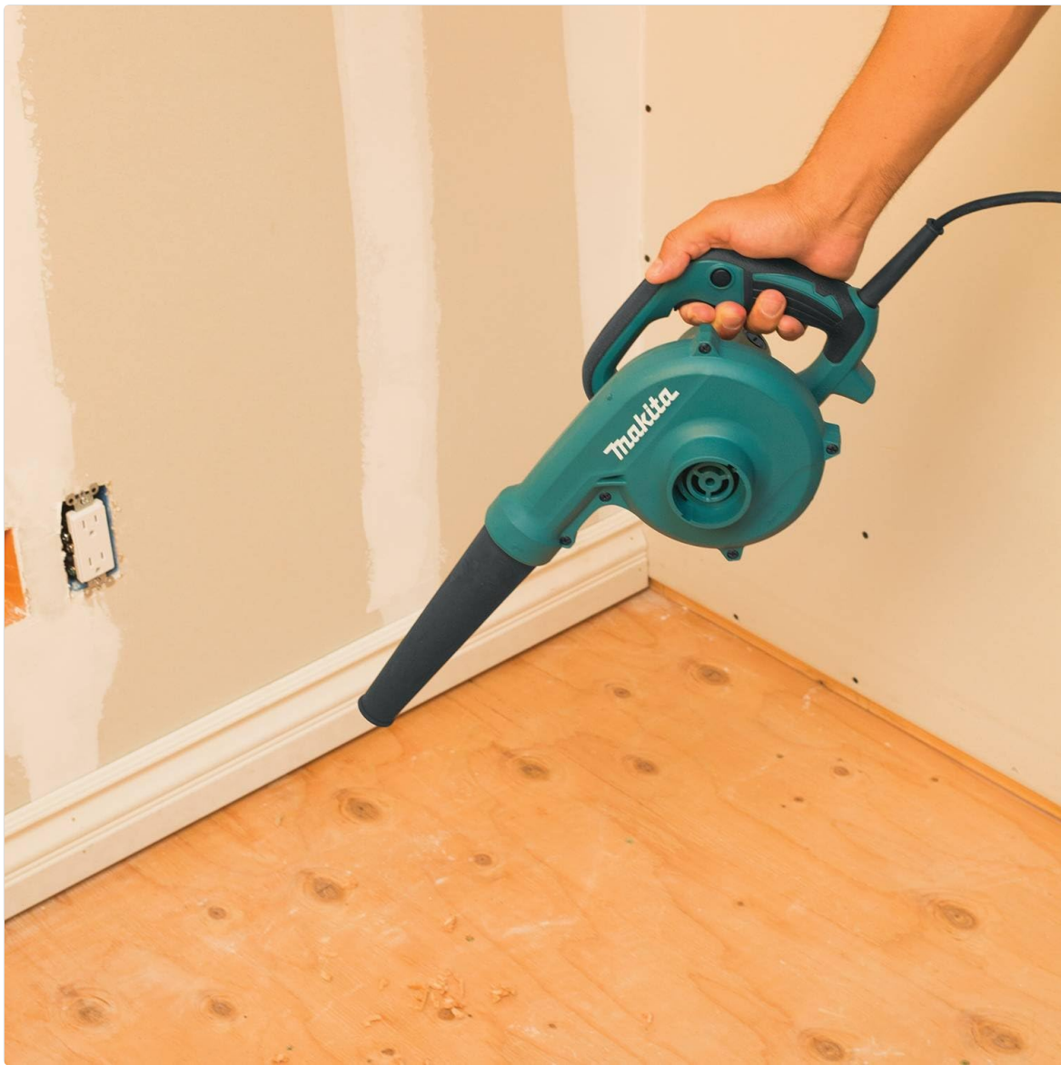
Figure 4.3: Demonstrating the blower in use to clear debris from a floor.
