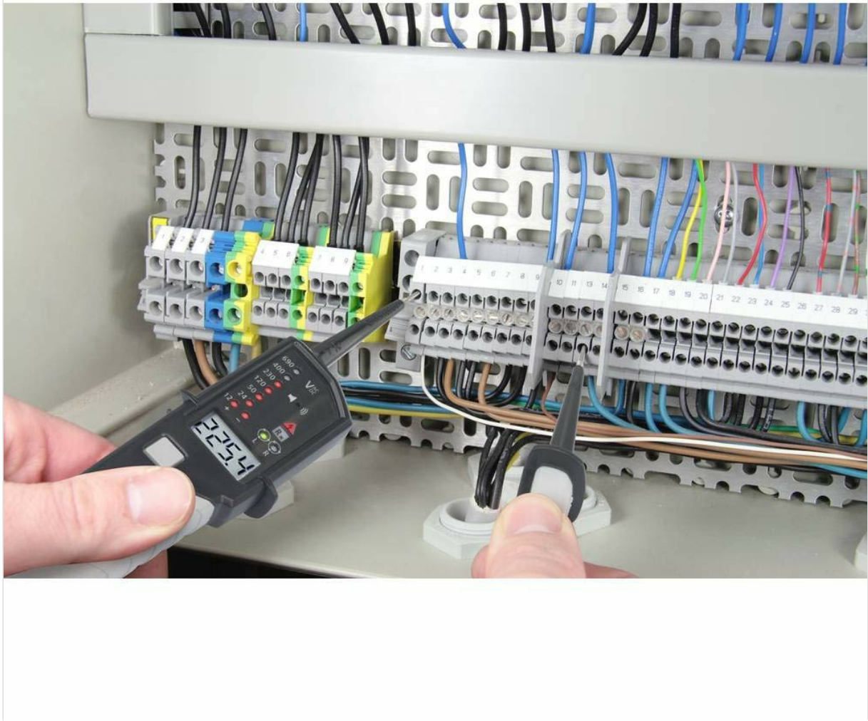
Figure 3: The VC-55 LCD tester actively measuring voltage within an electrical control panel, displaying readings on its screen.
