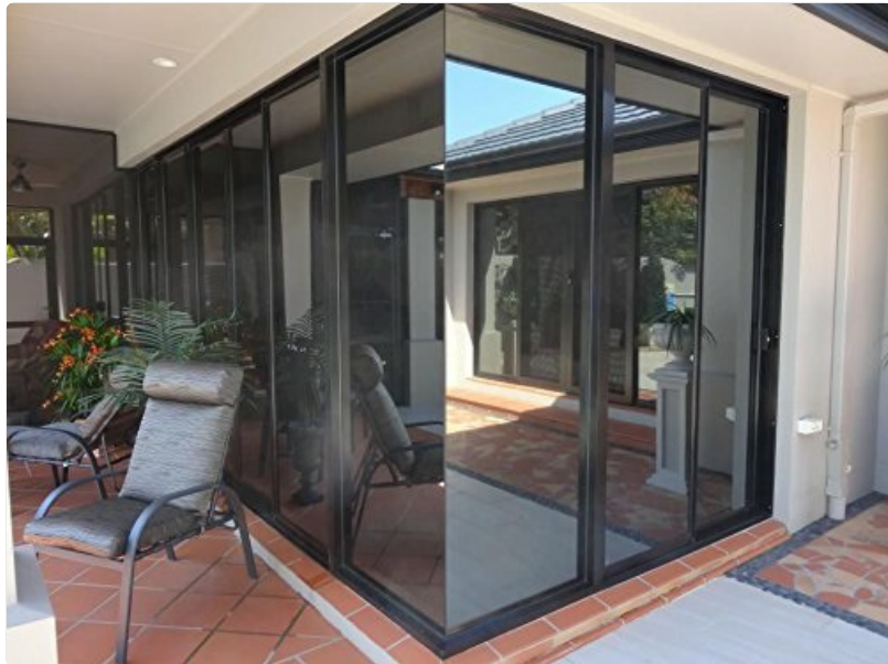
Figure 5.2: VViViD tint film applied to residential windows.
