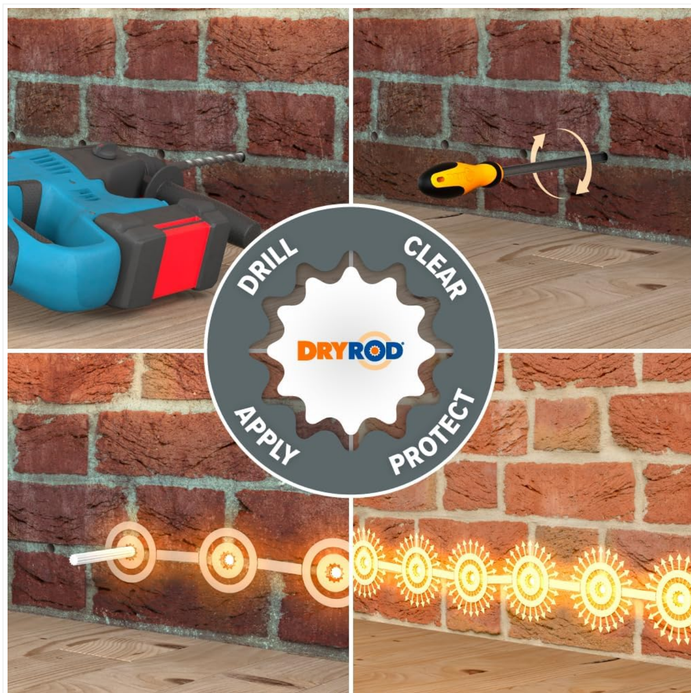
Figure 5: Illustration of rising damp and the effective barrier created by Dryrod treatment.
