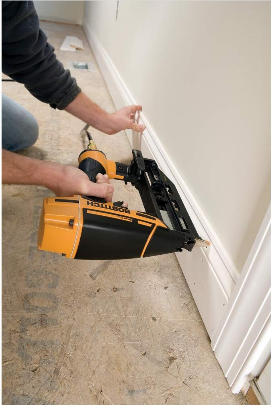
Image 5.2: Applying the nailer to secure baseboard, illustrating practical application.
