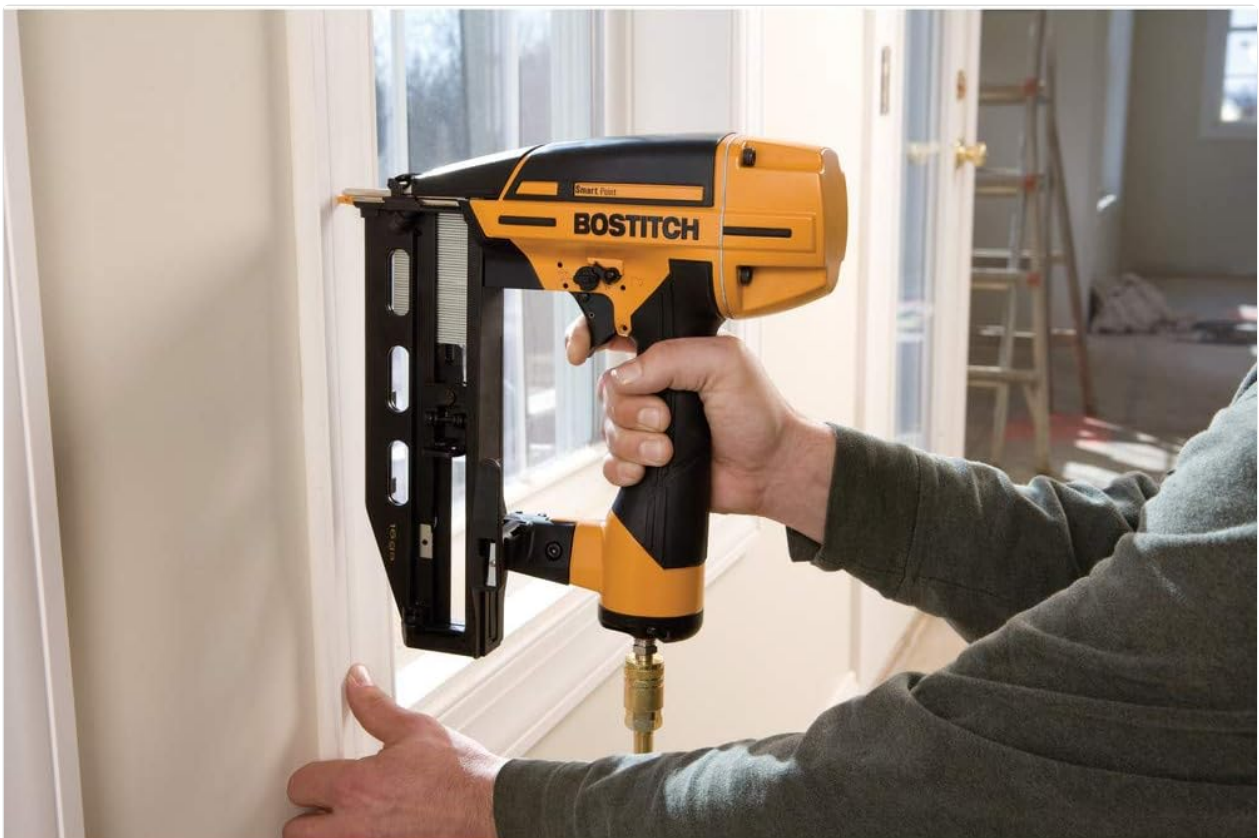
Image 5.1: Proper technique for using the nailer on door trim, demonstrating precise placement.
