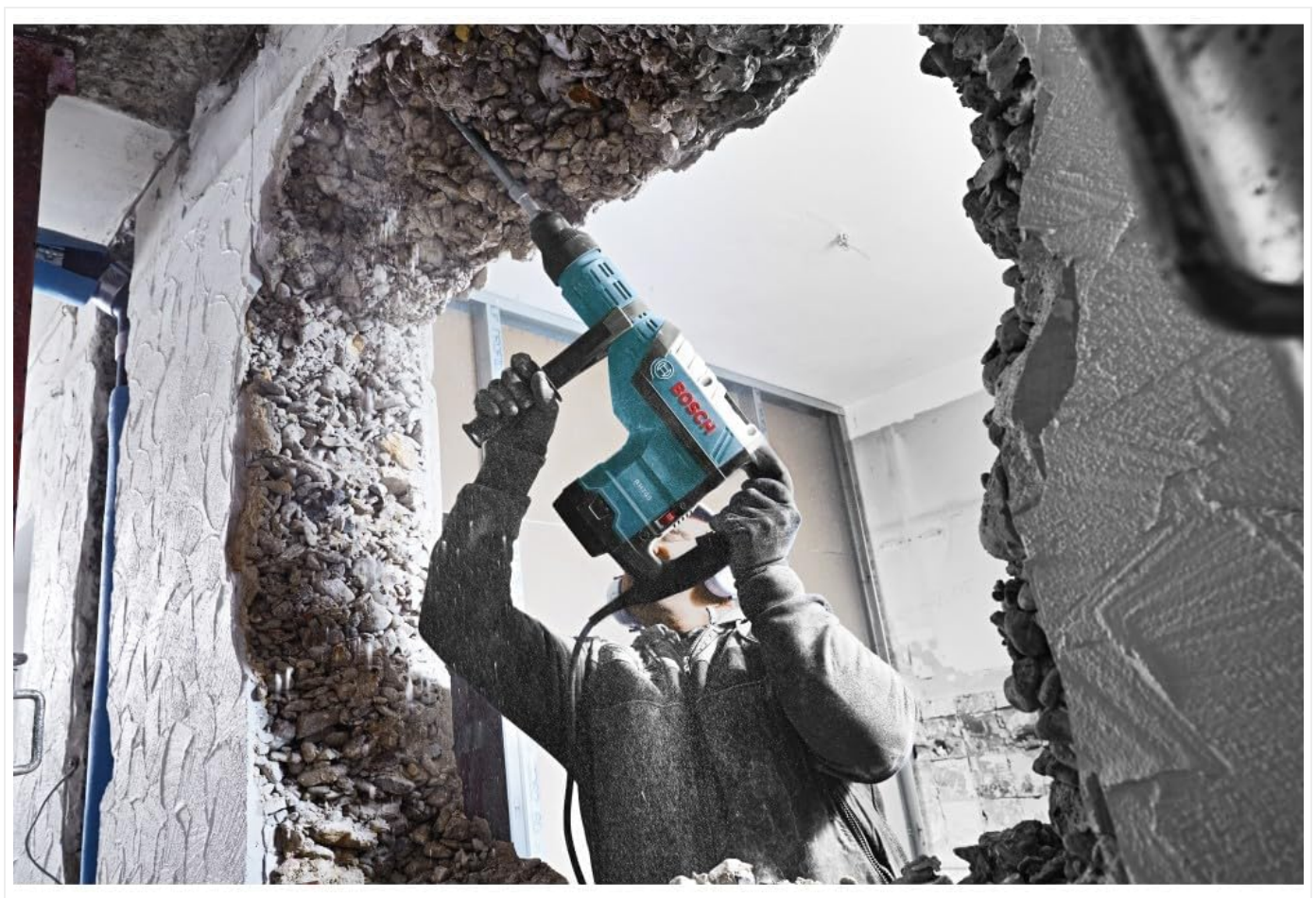
Figure 4: A worker performing chiseling work on a concrete wall with the Bosch RH745 rotary hammer. This illustrates the hammer-only mode in action.
