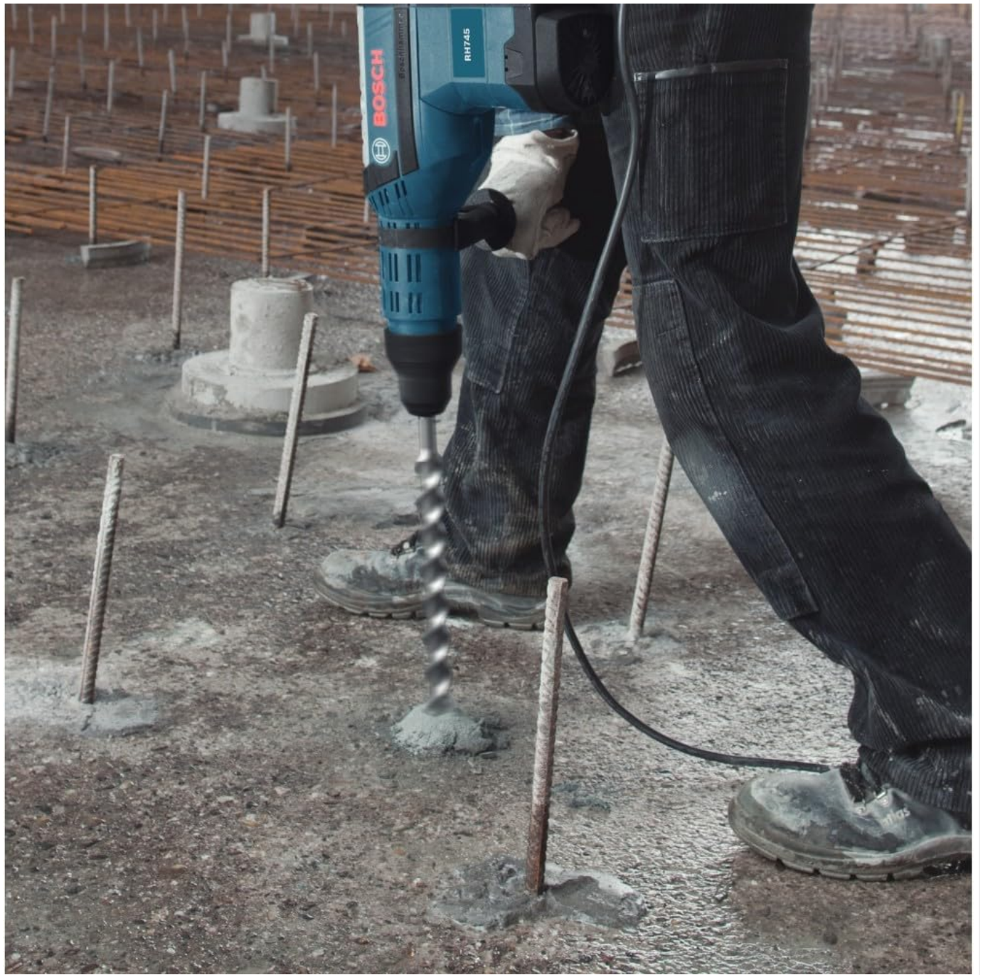
Figure 3: A worker demonstrating drilling into concrete using the Bosch RH745 rotary hammer. Proper grip and stance are shown.
