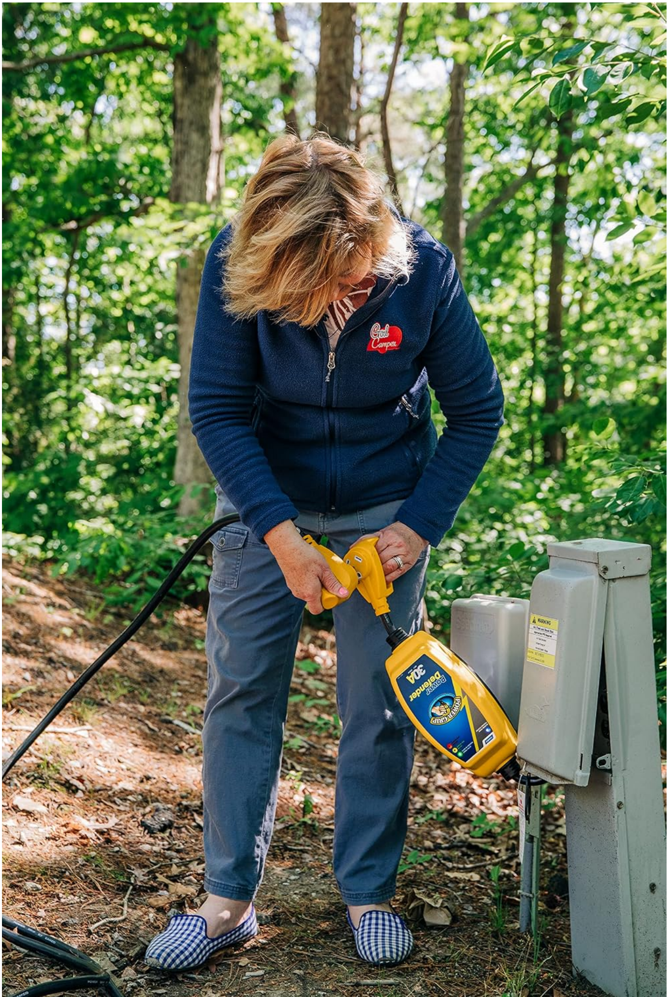
Image: A woman connecting the Camco Power Grip RV 30-Amp Voltage Protector to a campground power pedestal, demonstrating the ease of use with the Power Grip handle.
