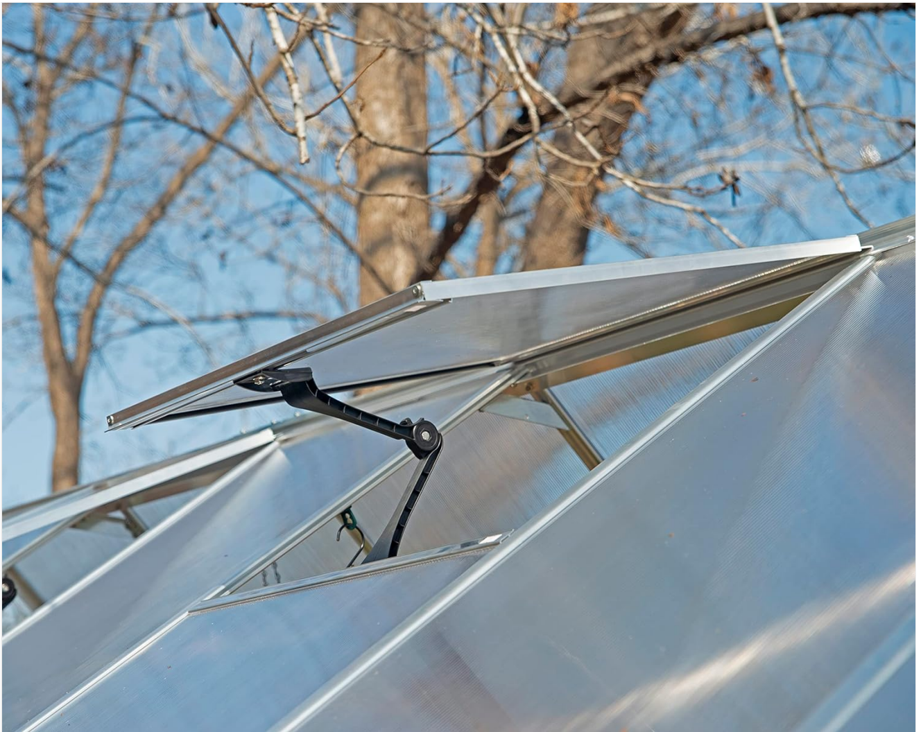
Image 3.1: Polycarbonate panel being inserted into the aluminum frame channel.
