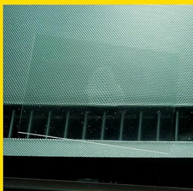
5 Remove apparatus & apply curing strip
