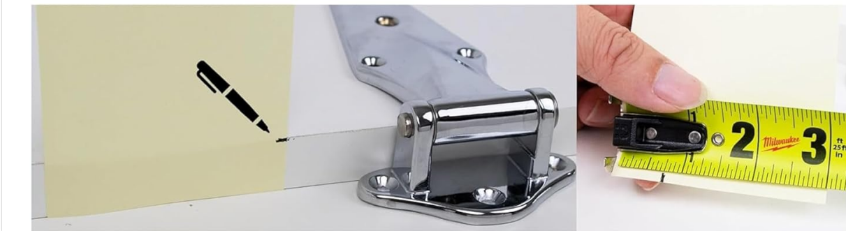
Figure 2: This image illustrates two methods for accurately measuring the offset required for latch installation: measuring the direct distance between the jamb surface and the door's height, and using a piece of paper to mark and then measure the offset height.
