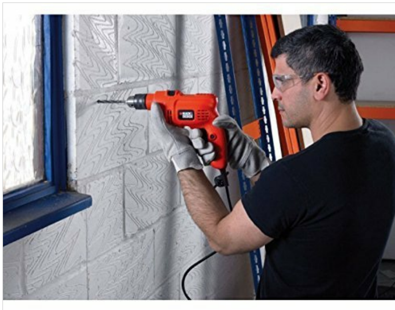
Figure 7: Example of drilling into a masonry wall.
