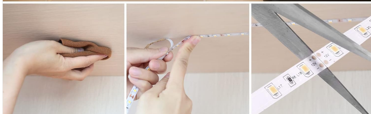
Figure 5.2: Installation Process: Clean surface, peel adhesive, and cut at marks.
