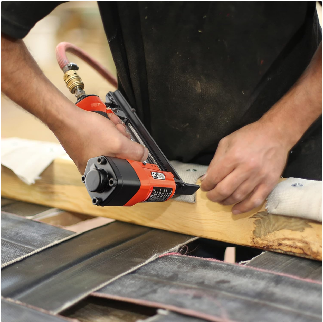
Figure 4: Stapling fabric to a wooden frame.
