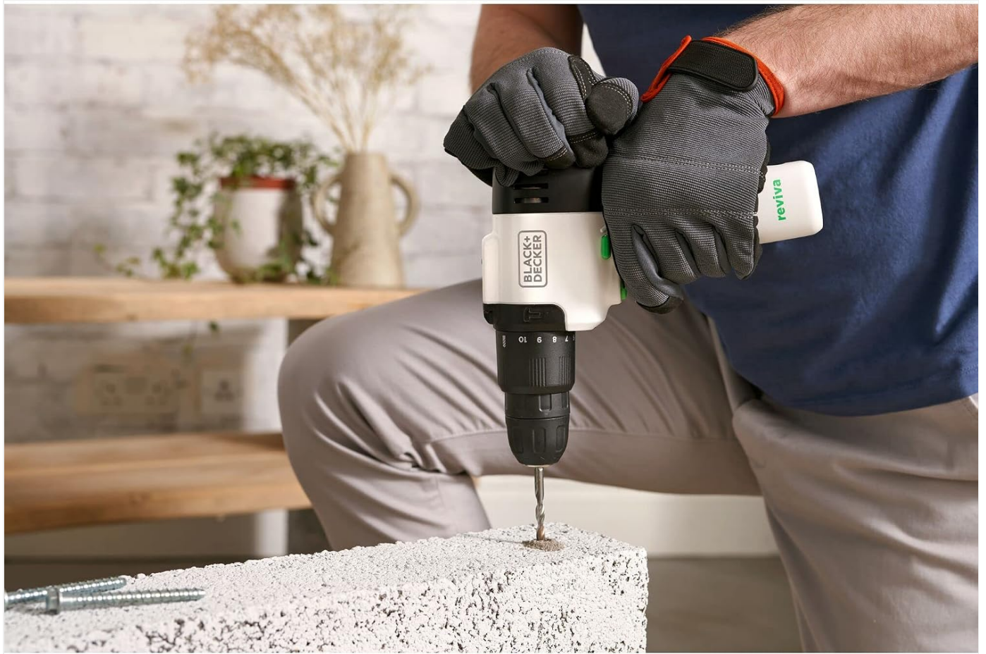
Figure 6: A user demonstrating the hammer drill in action, drilling into a concrete block.
