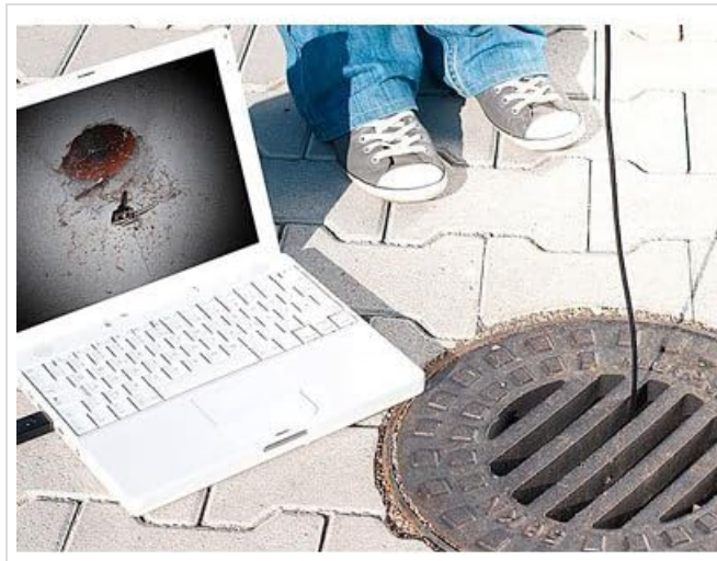
Image: The endoscope camera capturing a detailed view of a rusty object within a manhole, displayed on a laptop. This illustrates the camera's ability to provide clear visuals of internal structures.
