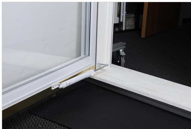
Image: The jamb bracket is securely attached to the door frame, ready for the closer.
