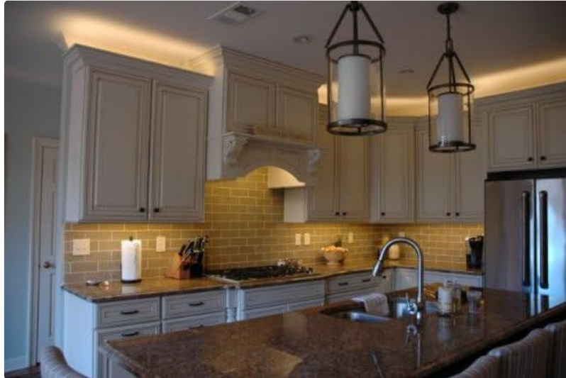
Figure 4.1: Example of LED strip installation for under-cabinet and above-cabinet lighting.
