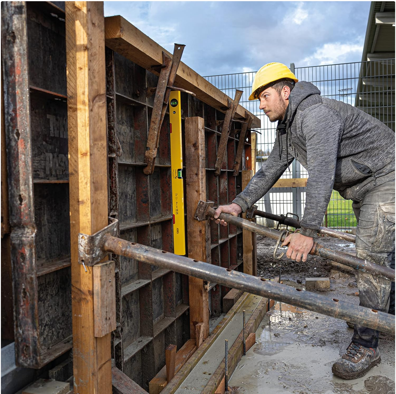
Image 4.1: A construction worker utilizing the spirit level for vertical alignment on a construction site.
