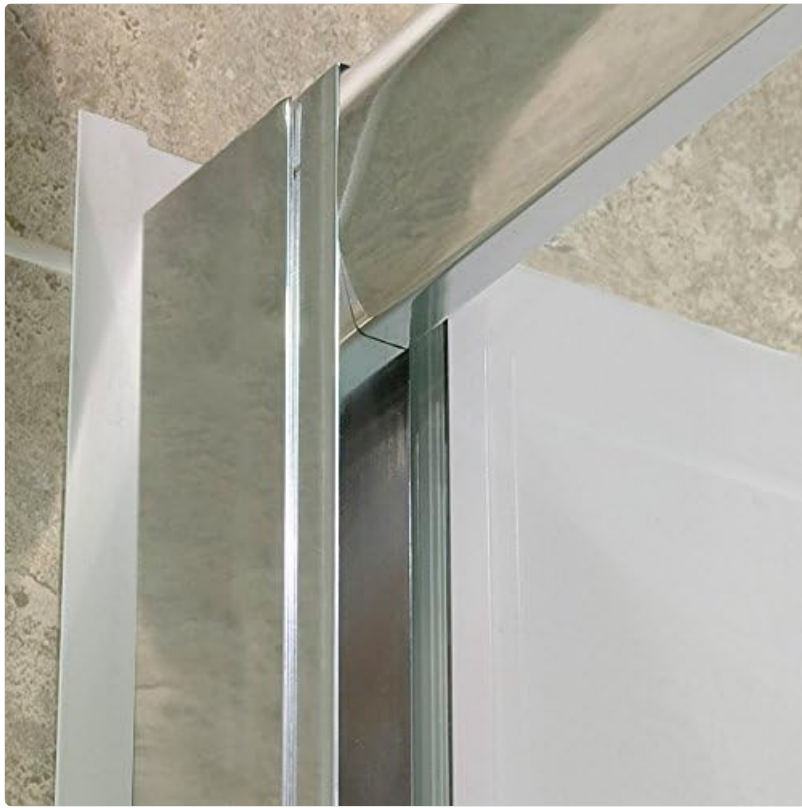
Figure 2: Installation of the bottom rail with sealant.
