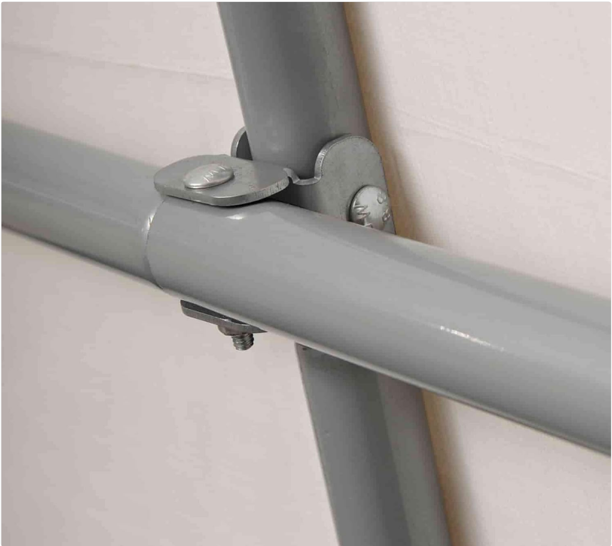
Image 4.1: Detail of the ShelterLock steel stabilizers, which enhance frame strength and stability.
