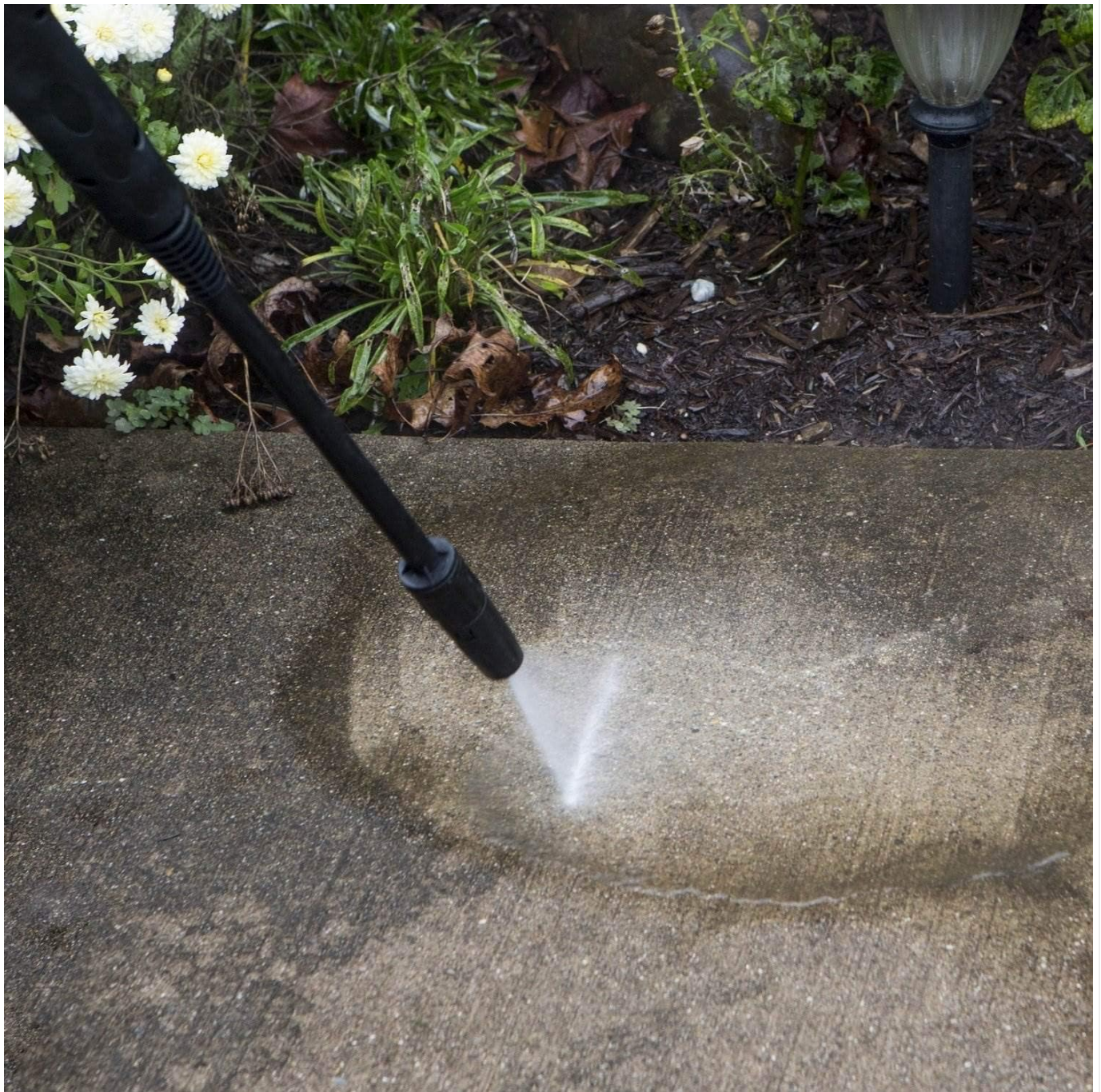
Figure 4.2: Cleaning a concrete surface with the pressure washer.
