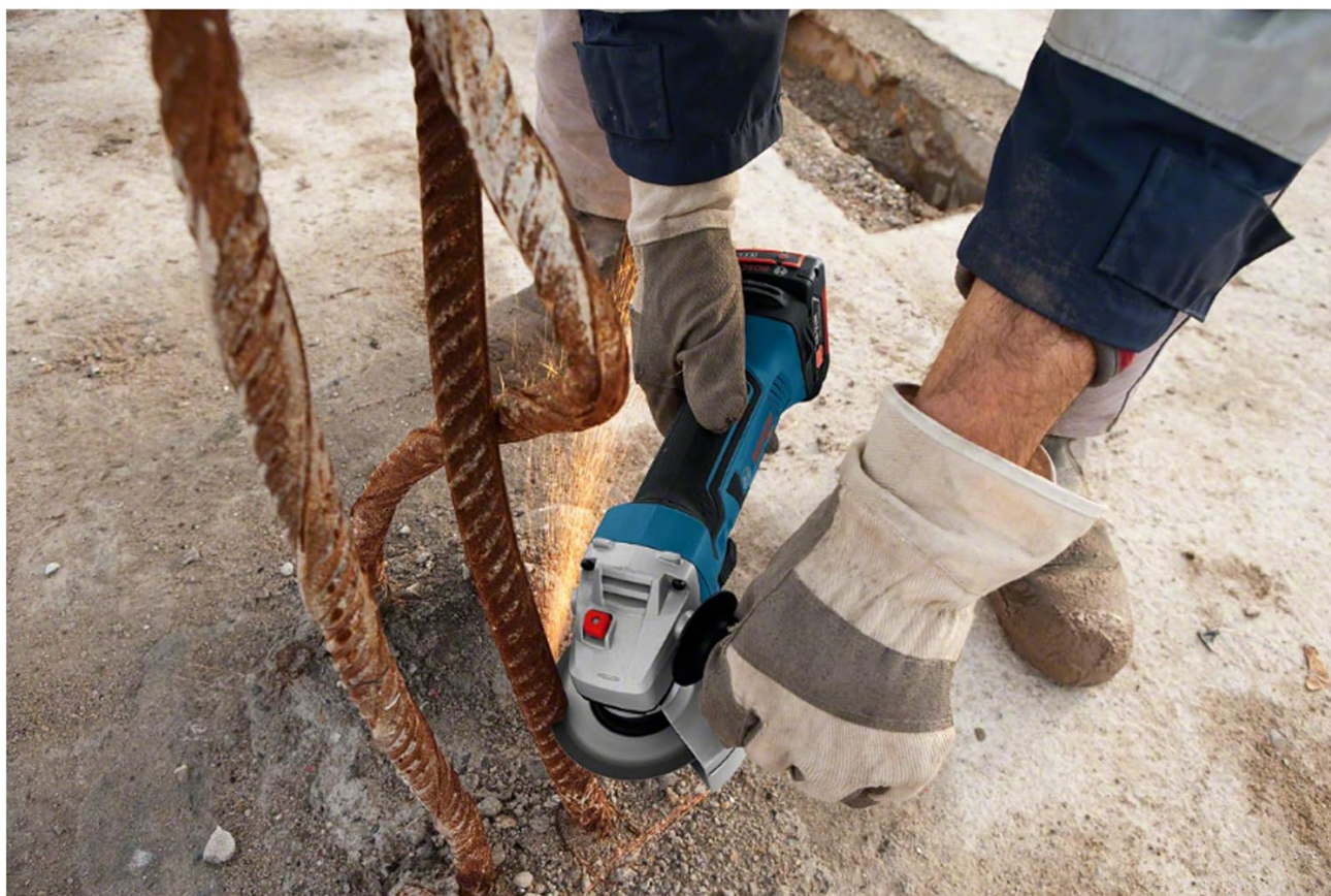
Figure 4: Angle grinder in use grinding rebar. This image shows the tool being used for grinding applications, generating sparks as it removes material from rebar.
