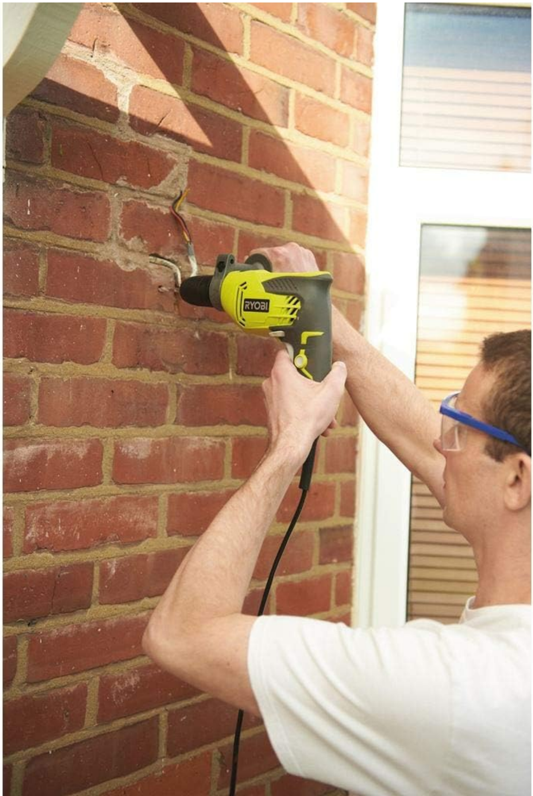
Image 5.1: A user demonstrating drilling into a wall with the Ryobi RPD500-G, wearing appropriate safety glasses.
