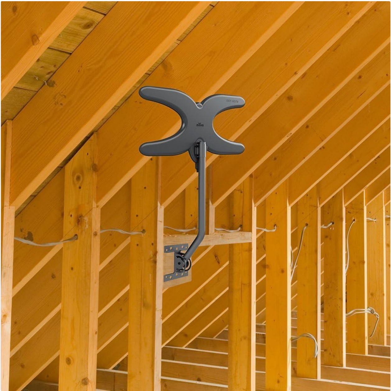
Image: The Mohu Sky 60 antenna installed on a rooftop, demonstrating an outdoor placement option.
