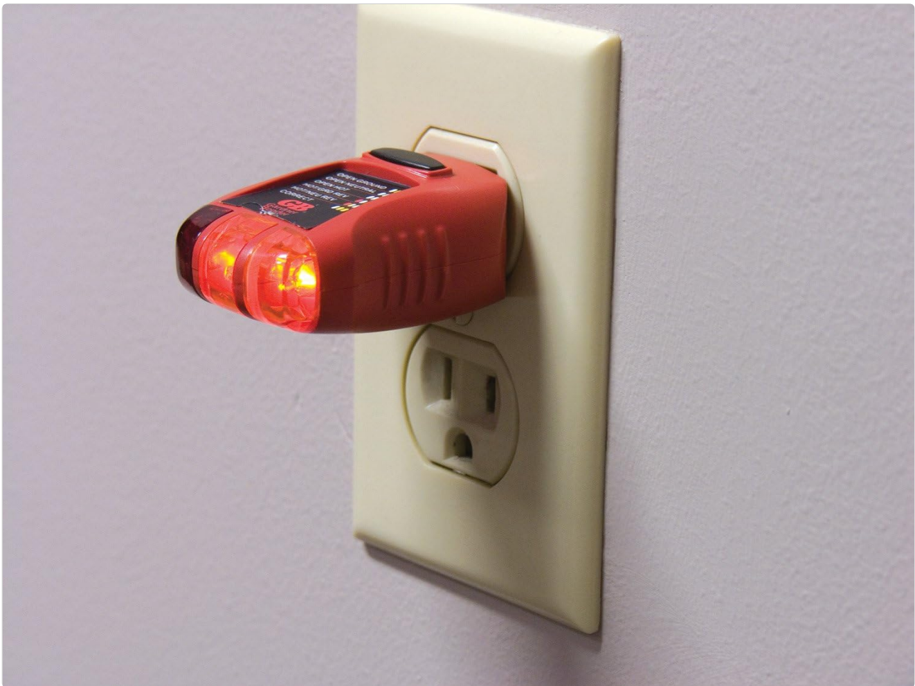
Figure 5: GFI-3501 plugged into an outlet indicating correct wiring.
